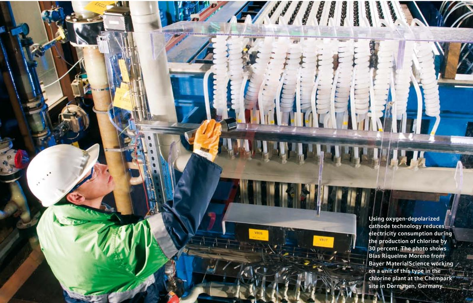
Using oxygen-depolarized cathode technology reduces electricity consumption during the production of chlorine by 30 percent. The photo shows Blas Riquelme Moreno from Bayer MaterialScience working on a unit of this type in the chlorine plant at the Chempark site in Dormagen, Germany.
